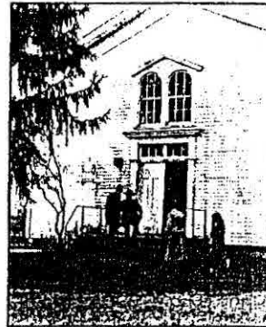
The Church in the village of Shirland holds services only on Thanksgiving and Memorial Day. Note the frontier costume.
